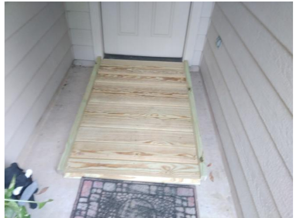
The completed ramp, with side guards attached.
