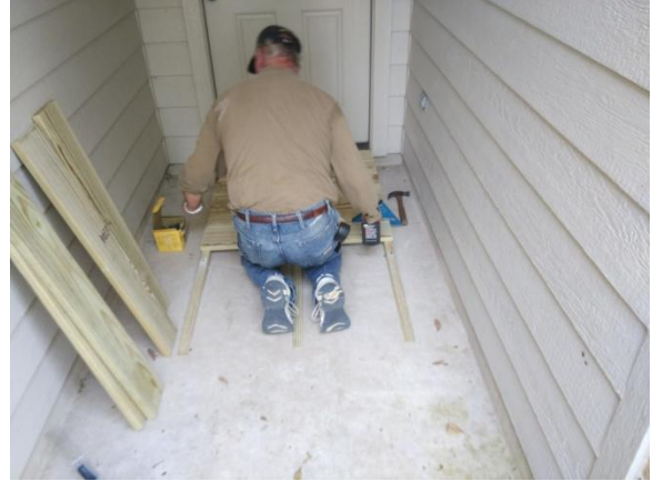
Construction of the front door ramp.
