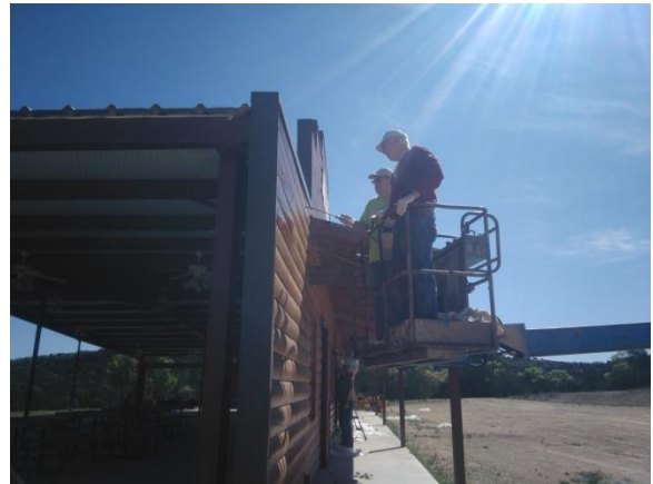
Keith sprayed the stain with a bug sprayer and Chuck smoothed it out. You can see the open pavilion where the women were busy painting the support poles.
